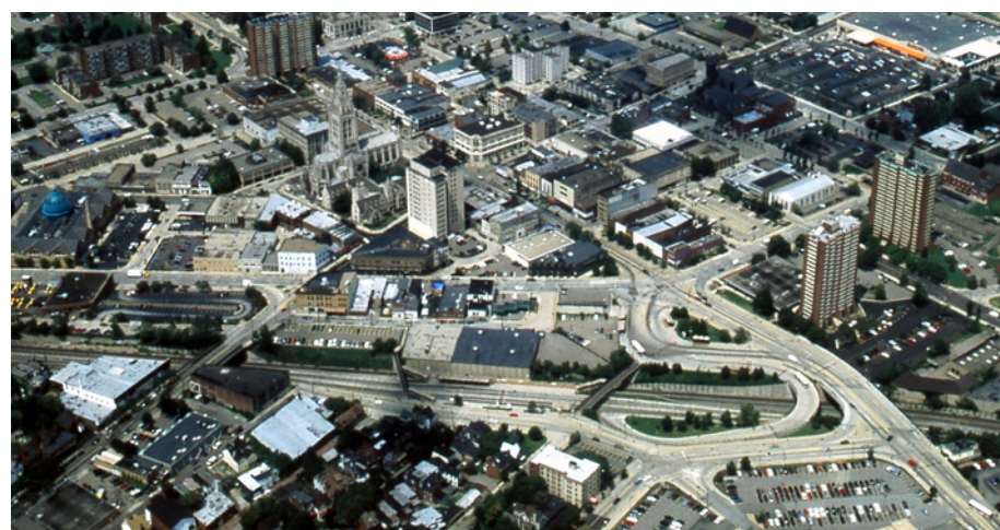
EAST LIBERTY, PITTSBURGH: Located on the East Busway, both its downtown and its neighborhoods are within walking distance of premium regional transit. New developments as well as re-developments are occurring in the area.
