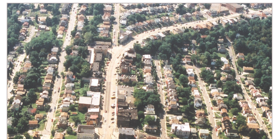
BEECHVIEW, PITTSBURGH: In Beechview, the LRT shares the road with cars. The LRT is a vital part of the community as it connects the surrounding neighborhoods to the commercial core. Beechview's streets are pedestrian friendly, connected and supportive of transit.
