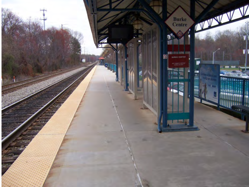
Fig. 8-1 Example Station and Platform (VRE Virginia)
