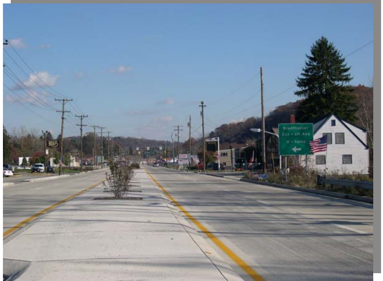
S.R. 22 B01 following construction
