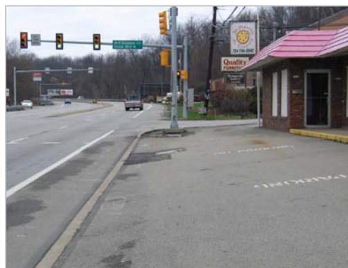
US Route 19 at Demar Road
