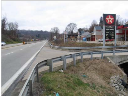
Right turn In/Out Only – No Left Turns
