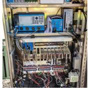
As part of this project, two intersections received new modern controller cabinet assemblies and audible emergency preemption systems. Global Positioning Satellite Antenna and Receivers were installed at the intersections to allow for timebased coordination during the weekday AM, Midday, and PM peaks as well as Saturday Midday Peak. Coordination of traffic signals is one of the most cost effective ways of improving traffic flow along a corridor.
