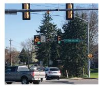
This project included the installation of Ethernet Radio systems to improve communications back to Cranberry Traffic Management Center. In addition, new LED pedestrian countdown signals and emergency vehicle preemption systems were install at some intersections to improve safety and improve emergency response times. Improvements have prepared the corridor for future responsive or adaptive signal operations.
