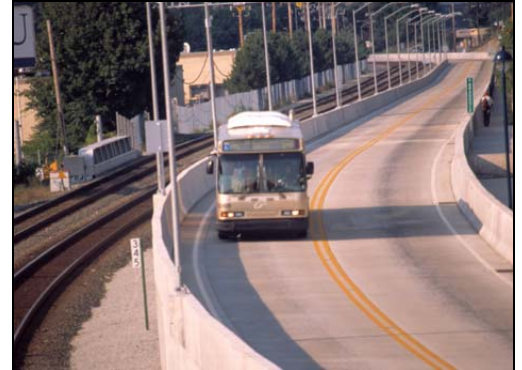
East Busway Extension near Roslyn Station
