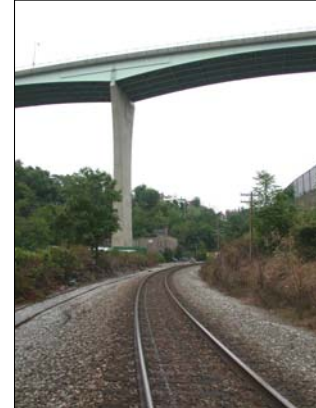
CSX ROW at Bloomfield Bridge
