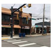
As part of this project, the Brownsville Rd and Marylea Ave intersection received a full signal replacement with ADA curb ramps. Global Positioning Satellite antenna and receivers were installed at the intersections to allow for time-based coordination. Coordination of traffic signals is one of the most cost effective ways of improving traffic flow along a corridor.
