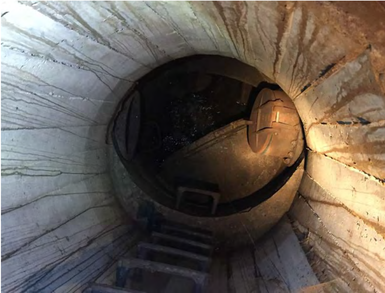
Figure B-29. Photo of MH-22 flap gate from survey
