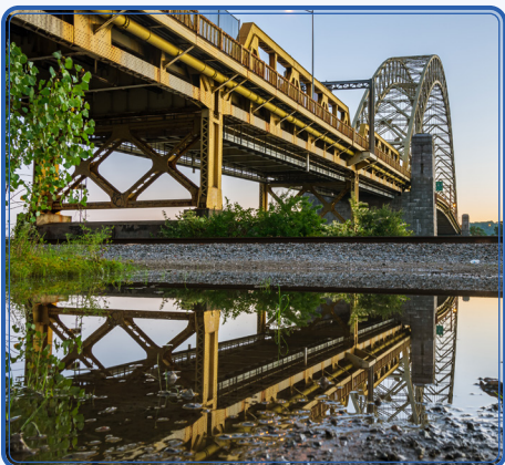
West End Bridge, City of Pittsburgh
