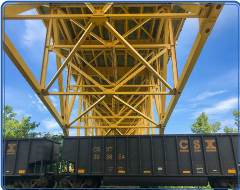
Under Donora Monesson Bridge, Westmoreland County
